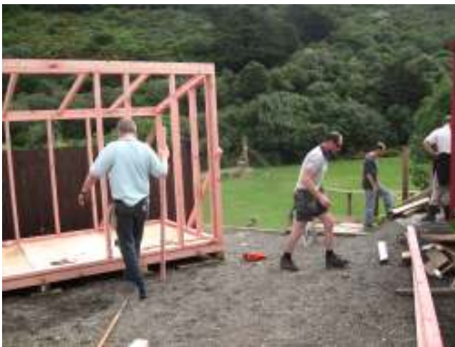
Building the hall storage shed
